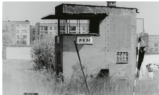
Photograph. Pyskowice Miasto railway station, disused PKM signal box awaiting demolition. From private archives and courtesy of A. Kaliszewski
